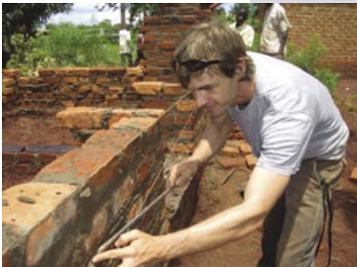
David Vimont points brickwork on a Habitat for Humanity construction site in Uganda.
