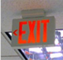
Exit signs are an excellent, low-cost, low-labor opportunity to increase the energy efficiency and safety of your facility. Replacing incandescent exit signs that operate at about 40 watts per sign, or fluorescent exit signs that operate between 12 and 20 watts per sign, with an [ENERGY STAR qualified exit sign](#) can
