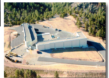
Aerial view of the Dual Axis Radiographic Hydrodynamic Test facility
