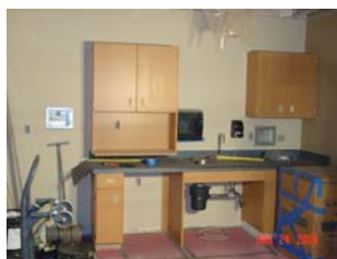
Kitchen facilities going in
