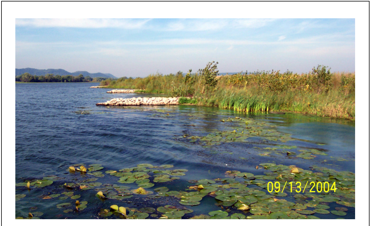
Figure 29: Constructed Islands with Sacrificial Berms, Rock Groins, and Native Vegetation, Upper Mississippi River NW&FR
