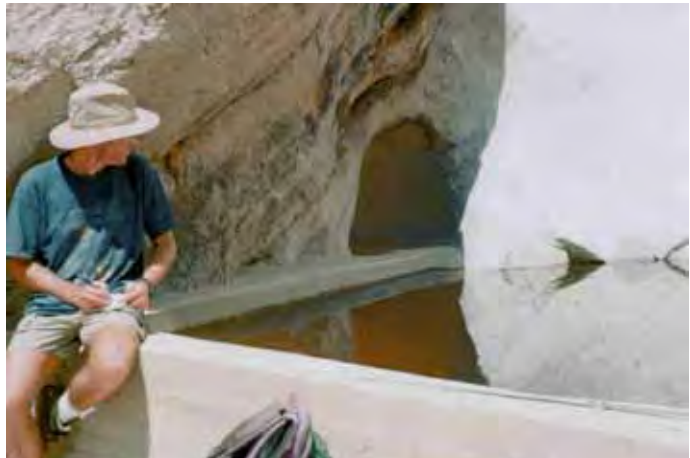
Dam at Heart Tank- this developed structure increases the capacity of Heart Tank, a natural tinaja
