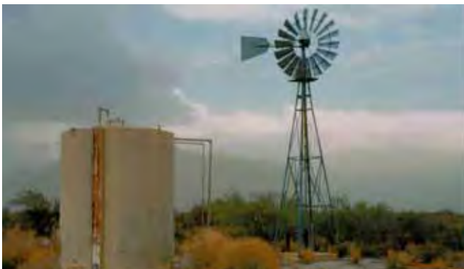
Papago Well and water storage tank
