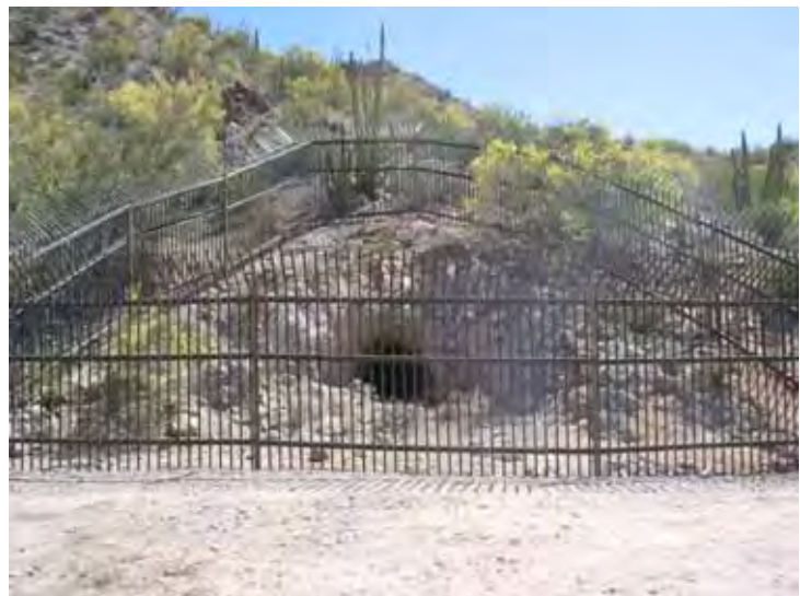
Fence around entrance to lesser long-nosed bat maternity roost Photo by Curtis McCasland
