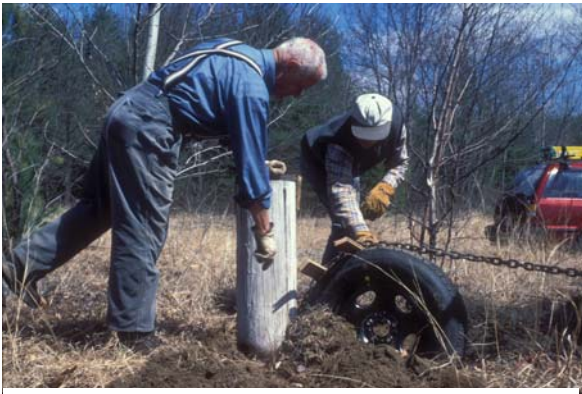
Volunteers removing the former obstacle course: Photo by Marijke Holtrop
