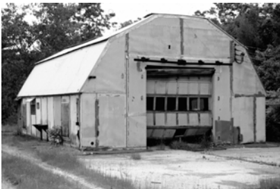
One of the buildings that has been removed from Assabet NWR: Staff photo
