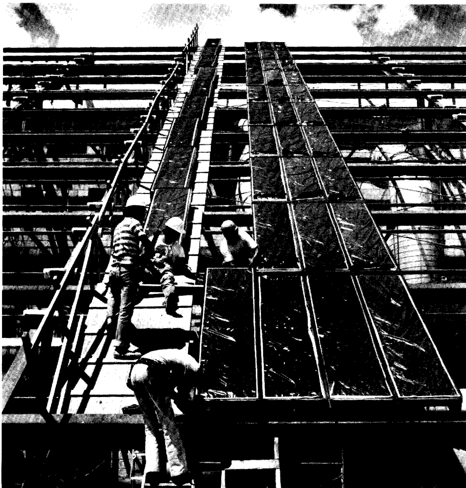
Harold spearheaded the drive for the Laboratory's National Security and Resources Study Center, shown here under construction in 1976.
