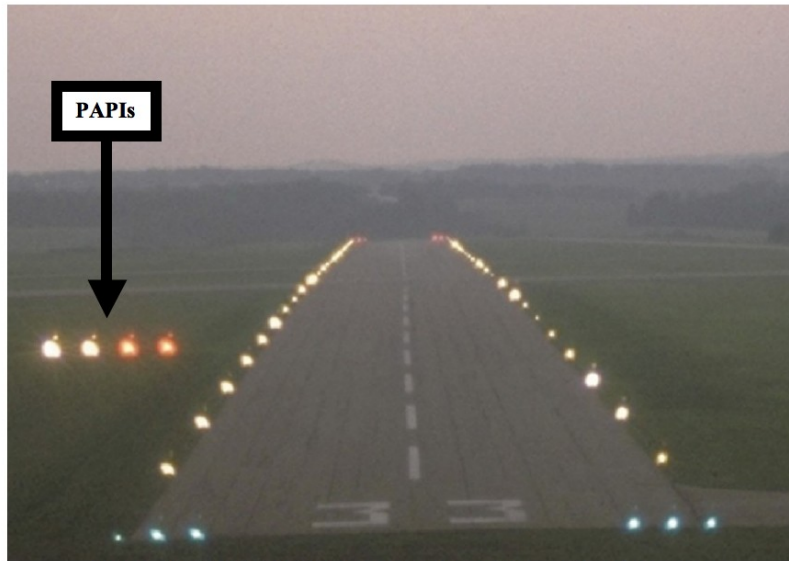
Figure 3. PAPI Light Fixture showing glide path information
