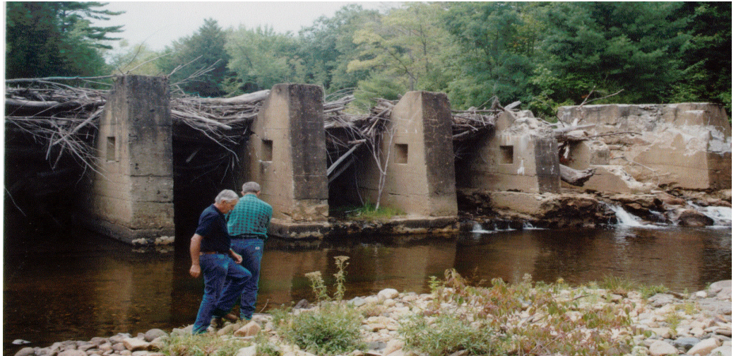
Bearcamp River Dam, Tamworth NH
