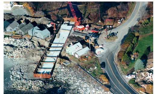
Culvert installation at Little River Salt Marsh
