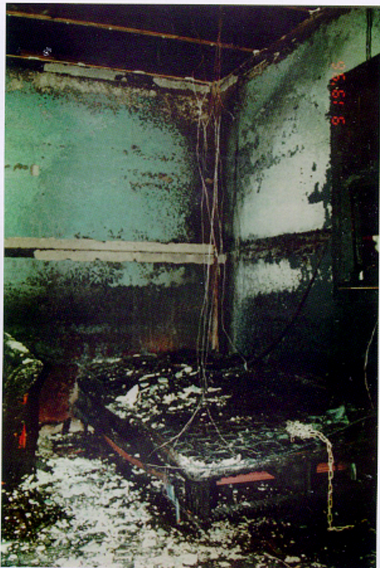
FIGURE 52. Photograph of the condition of the bed mattress and frame, Experiment 3.
