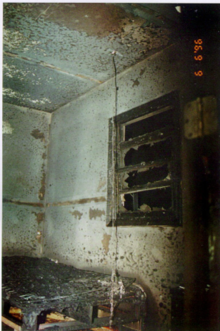
FIGURE 42. Photograph of the window and surrounding wall. Experiment 2.
