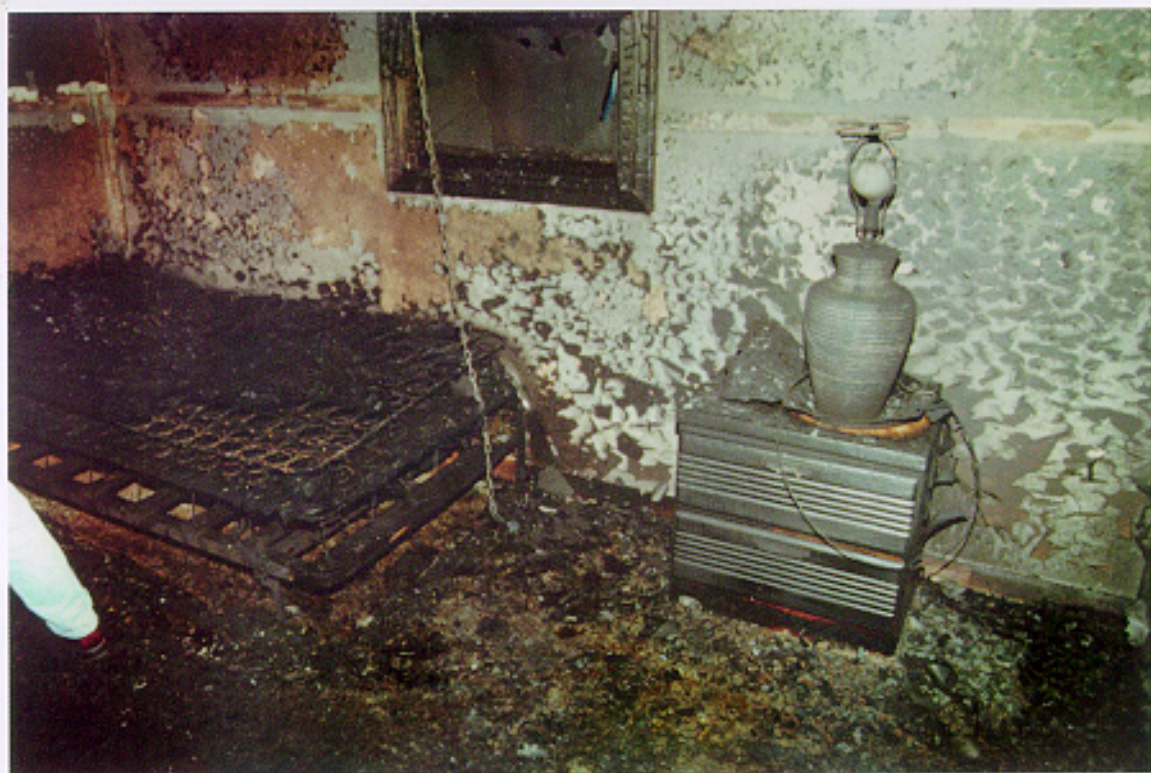
FIGURE 41. Photograph of the window and surrounding wall. Experiment 1.
