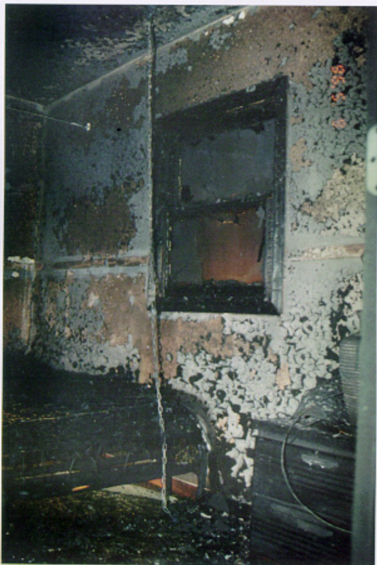
FIGURE 40. Photograph of the window and surrounding wall. Experiment 1.
