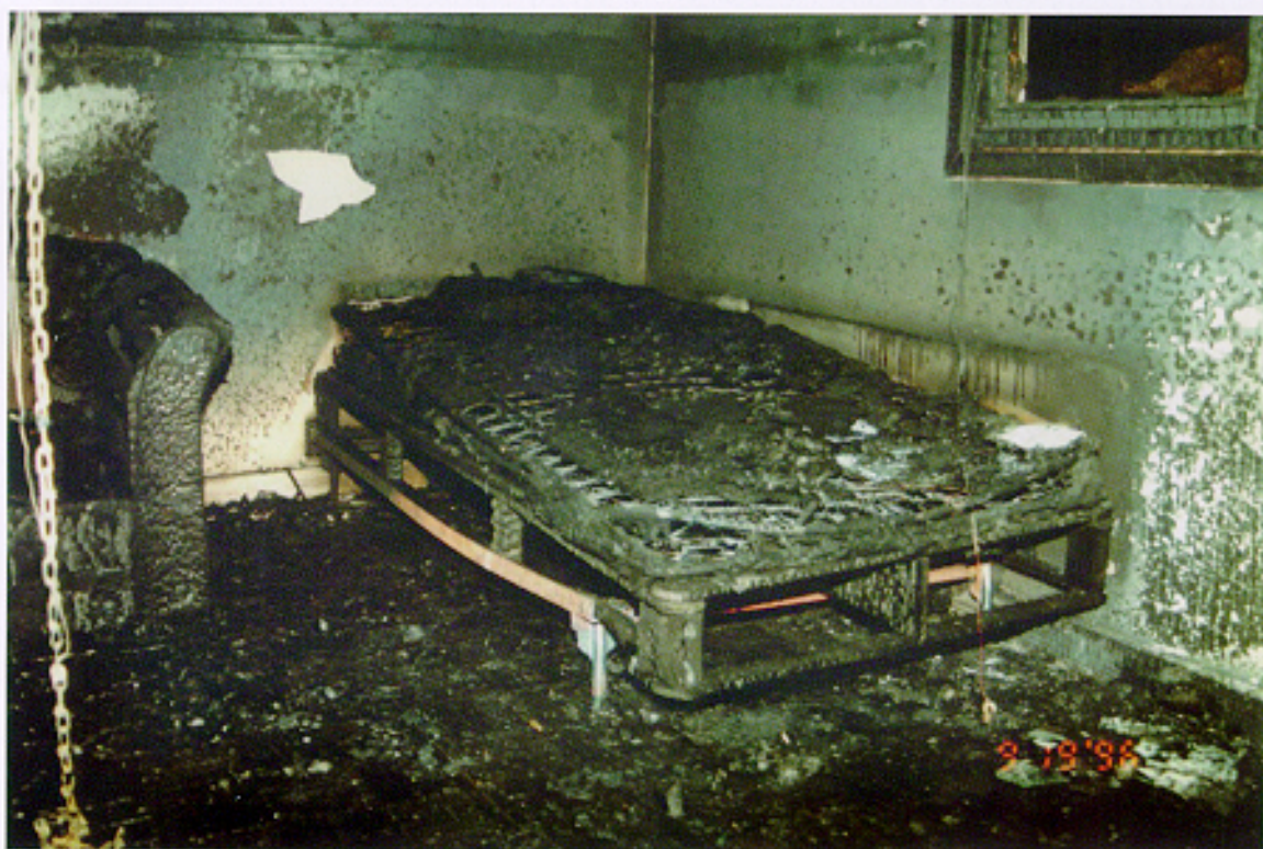
FIGURE 55. Photograph of the bed showing bed frame deformation. Experiment 4.
