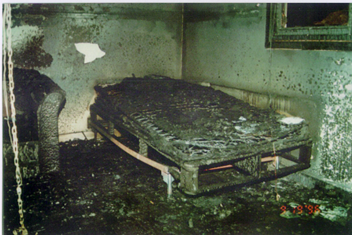
FIGURE 53. Photograph of the condition of the bed mattress and frame. Experiment 4.
