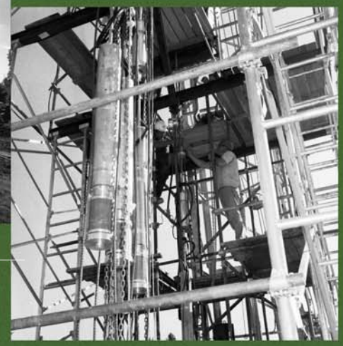
*** Dean List lowered canisters of SNL instrumentation 4,600 feet down into a drilling hole designed to measure the shock waves of the explosion.
