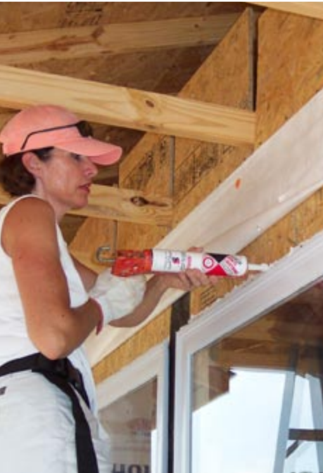
(left) Thorough air sealing and locating ducts in conditioned space are two ways the Loudon County Habitat affiliate improves the efficiency of its homes. Photo courtesy of Linda Morrison of Loudon County Habitat for Humanity.
