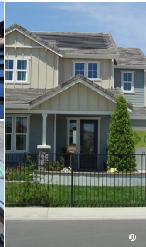
(photo series, continued) Cement tile system step-by-step installation
