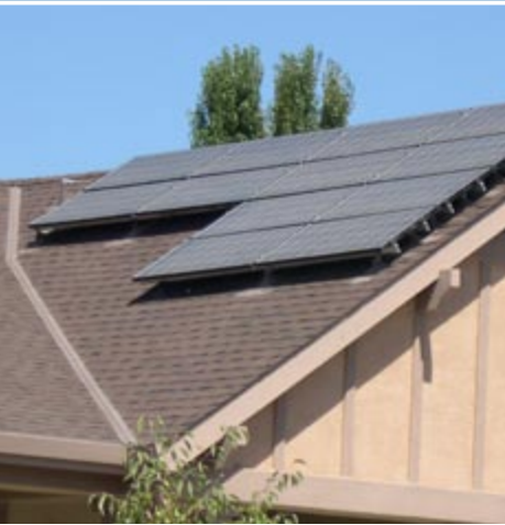
Clarum is building four zero energy research homes at Borrego Springs, California. Photos courtesy of Clarum Homes.
