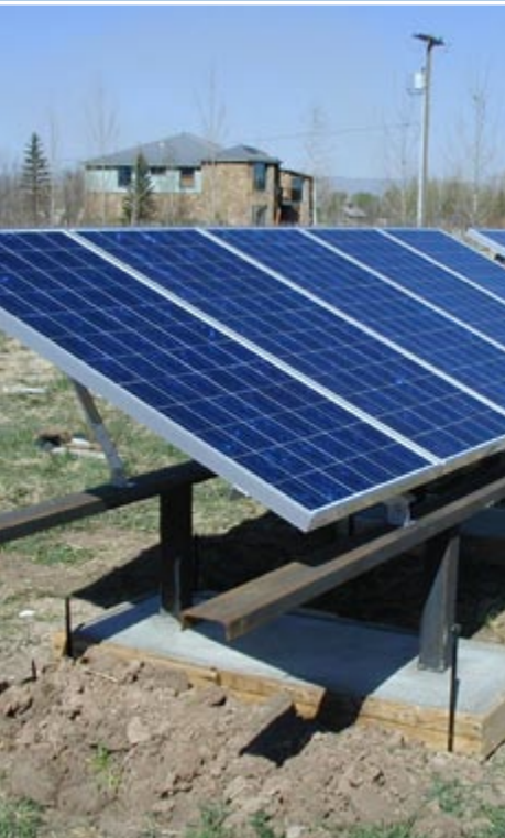
Ground mounts imbedded in concrete. Photos courtesy of Leif Juell, Alternative Power Enterprises, Inc.
