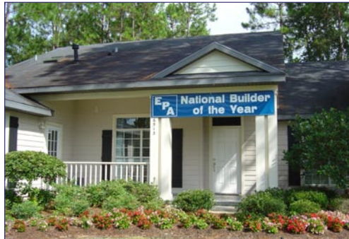
Atlantic Design, a Building America partner, was recognized as a 2000 EPA Builder of the Year for its quality energy-efficient construction.
