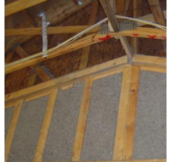
Blown-in wall insulation
