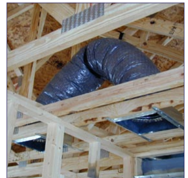
FIGURE 19: Jump Ducts
