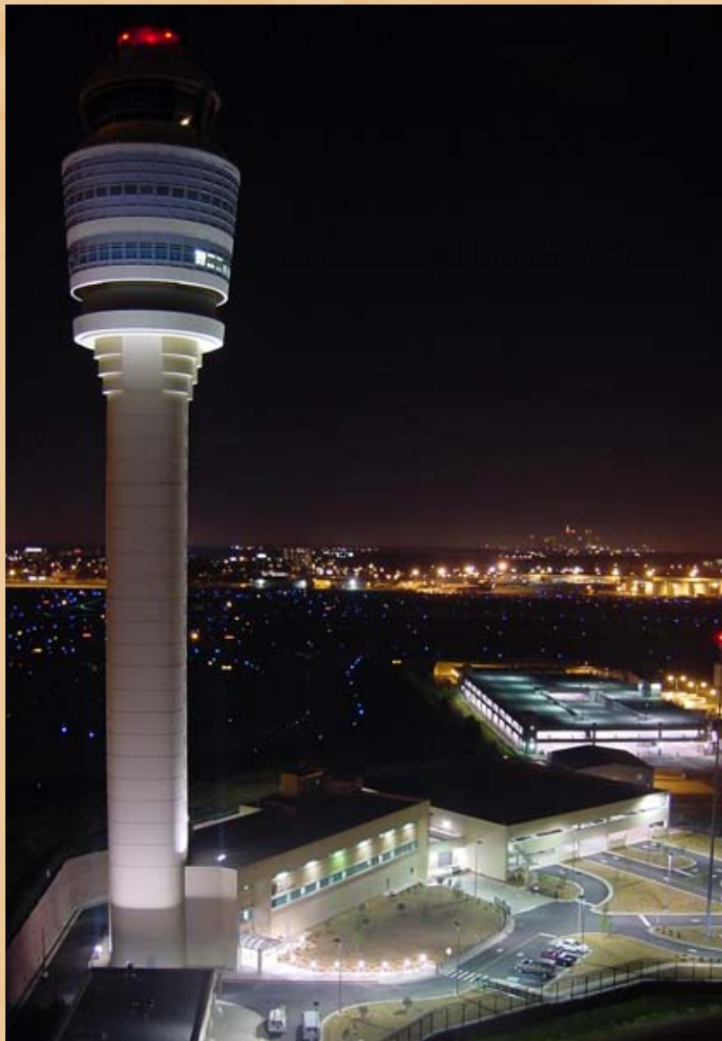
State-of-the-art air traffic control towers, like this one at Hartsfield-Jackson Atlanta International Airport, are helping air traffic controllers better guide current air traffic as well as accommodate future growth, making the safest aviation system even safer. Credit: Greg Haire, Airway Transportation System Specialist, Technical Operations, Hartsfield-Jackson Atlanta International Airport
