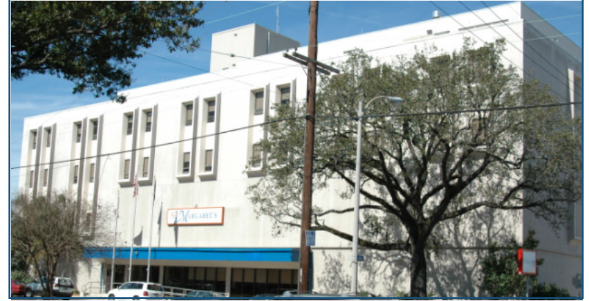
AFTER: Debris was removed and renovations were done to the Bywater Hospital to serve as St. Margaret's temporary facility. Source: FEMA Photos
