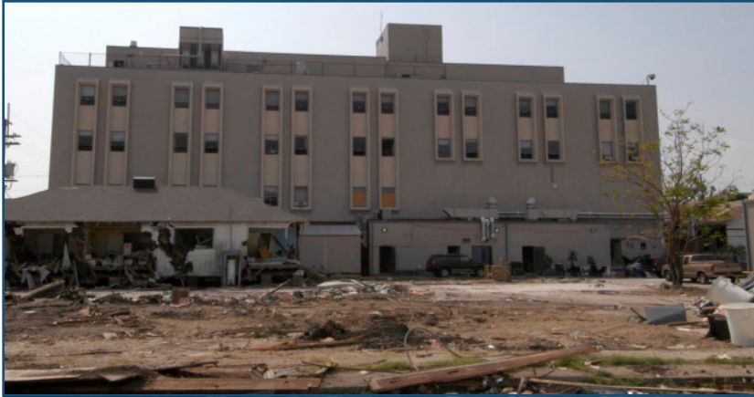
BEFORE: The hurricane caused damage to the Bywater Hospital building, which is located in a neighborhood near the nursing home. Source: FEMA Photos
