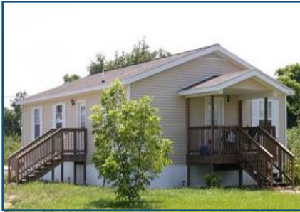
Ms. Ingraham's newly rebuilt home sits on in her hometown of Port Sulphur. Source: FEMA photos
