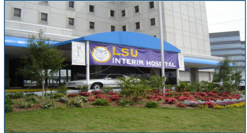
AFTER: FEMA assisted LSU with establishing a temporary hospital facility while final decisions are made about the future of the Medical Center of Louisiana at New Orleans. Source: FEMA Photos
