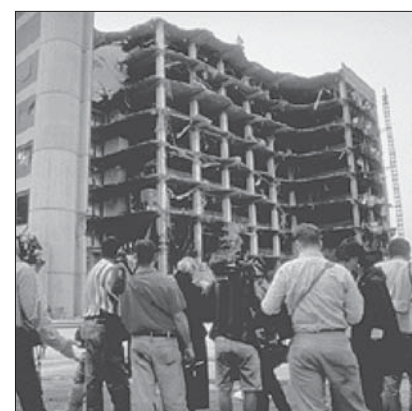
SNL is raising construction standards to produce structures that can better withstand a wide range of threats. In the Oklahoma City bombing, most of the victims were killed not by the blast but by the building, when its nine floors collapsed like a house of cards.
