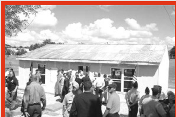
Building Success: Dignitaries from the United States and 34 Latin American and Caribbean countries inspect the composite building constructed using technology and funds from the U.S. Navy. The exterior of the building can be finished with any type of building material—such as brick, cement, or shingles.
