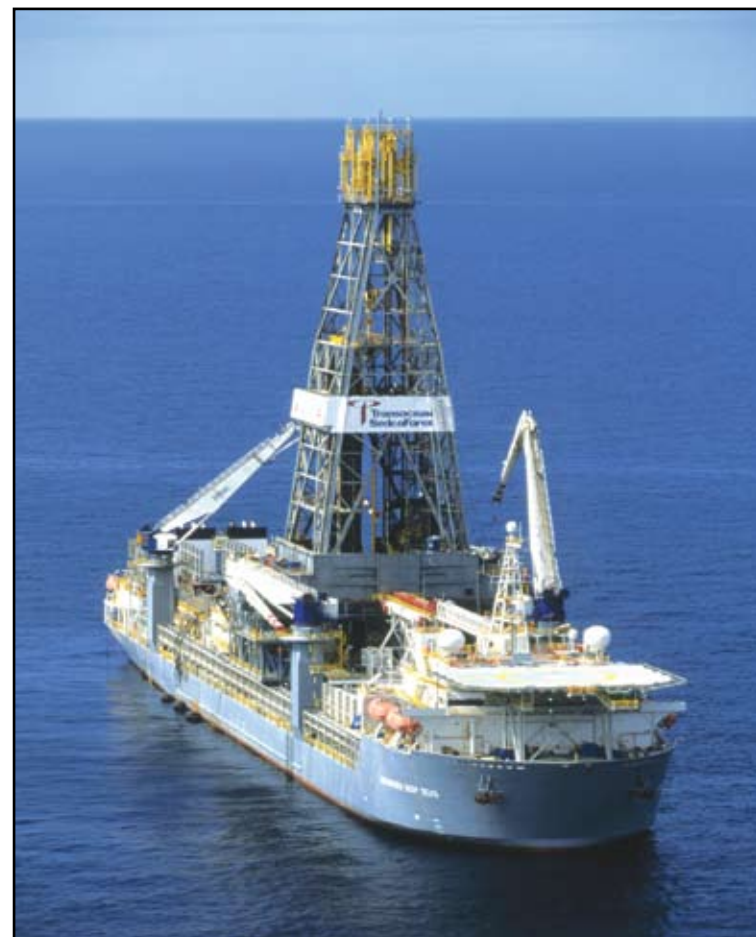
LANL's industry partner, Chevron Texaco, and its partner, Transocean Inc., achieved an industry record when Transocean's drillship, Discoverer Deep Seas, used LANL technology to drill Tonga, the deepest well ever drilled in the Gulf of Mexico, at a total vertical depth of 31,824 feet.
