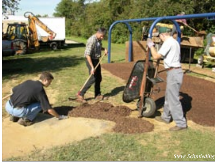
FPL researcher Ted Laufenberg (center) shows Bob Zeager (kneeling left) and Ted Illjes, both of Zeager Bros., how the stabilized wood fiber can be used to create a wheelchair-friendly path.
