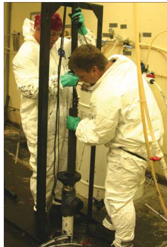
KSC's EZVI injection tool being lowered into the injection well.
