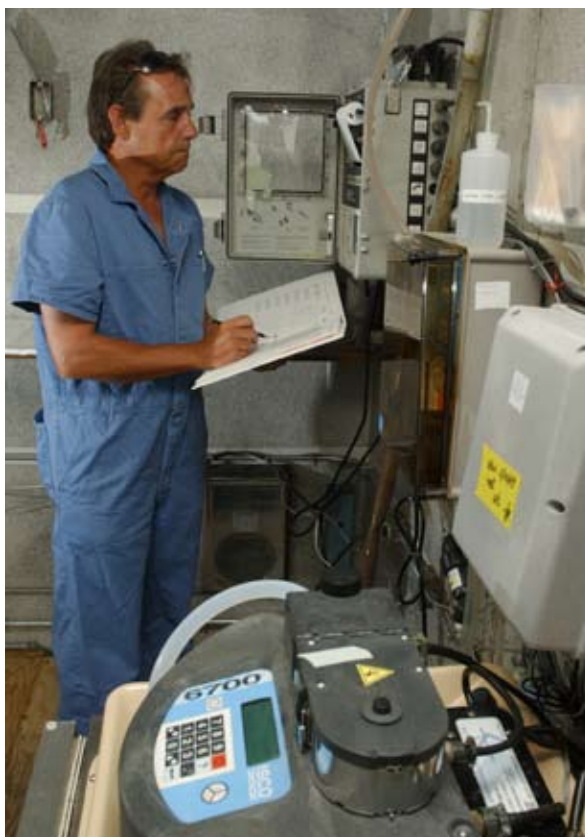
Y-12 environmental technician Mike Elliott performs maintenance and calibration tasks at a SWHISS Station.
