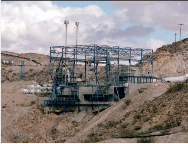
The test stand will enable indepth research leading to the development of long life-cycle rocket engines.
