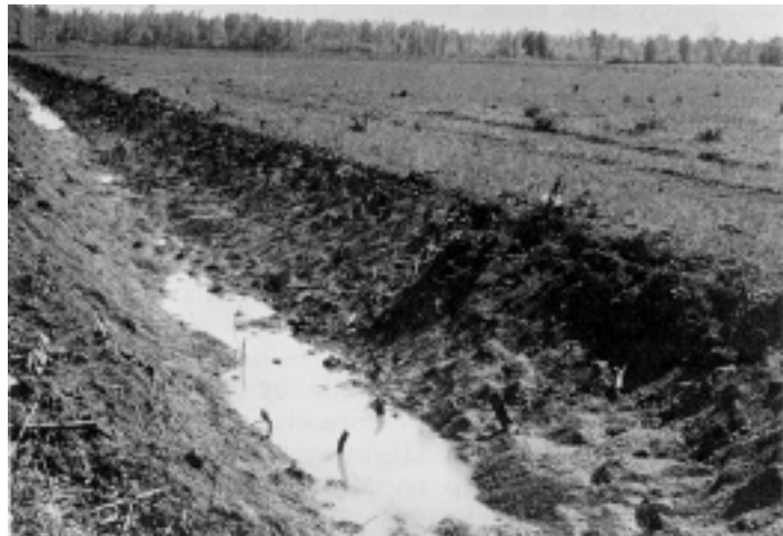
Figure 4.—Lateral ditch constructed to remove excess water.
