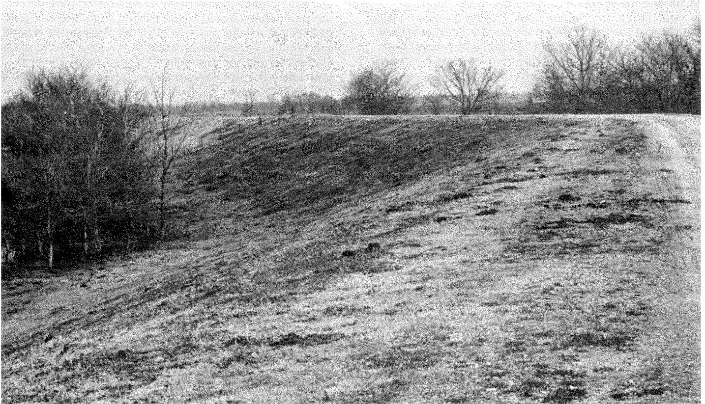
Figure 1.—This large earthen levee is part of a complex flood control system that protects a large part of south Louisiana from flooding by the Mississippi, Red, and Atchafalaya Rivers.
