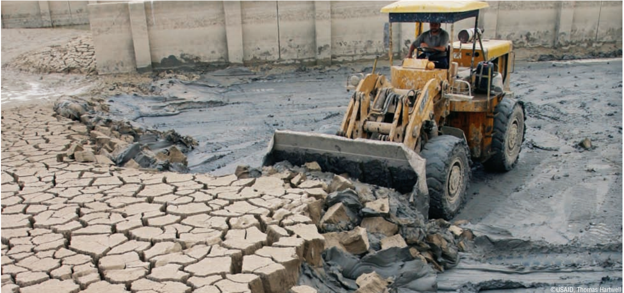
Loaders remove accumulated silt from storage reservoirs in the Sweet Water Canal IRRF project that supplies all the fresh water to the city of Basra and environs.
