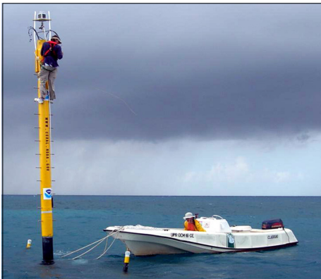
Jeff Absten installs electronics in the uppermost chamber of the new CREWS station in La Parguera, Puerto Rico perched about 17 feet above the ocean surface.
