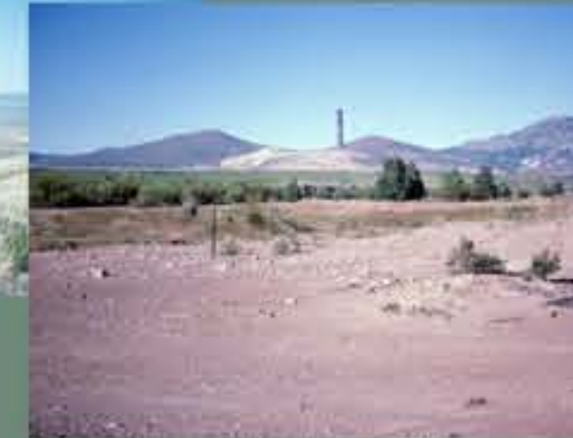
Site conditions north of chimney, 1997
