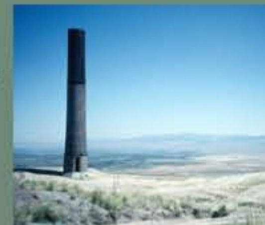
Washoe Reduction Works Chimney, 1999
