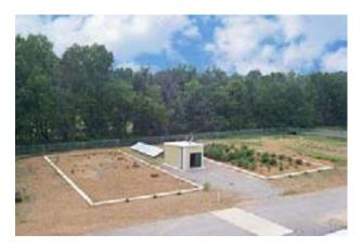
TVA has developed and patented (U.S. Patent No. 5,863,433) a novel subsurface-flow constructed wetland system—ReCip—in which vastly improved wastewater treatment is possible.
