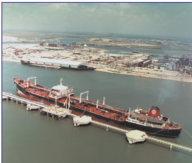
A tanker offloading Strategic Petroleum Reserve oil into a storage area along Gulf coast. Storage areas reduce the Nation's vulnerability to a shortage of petroleum in the event of a severe supply disruption.
