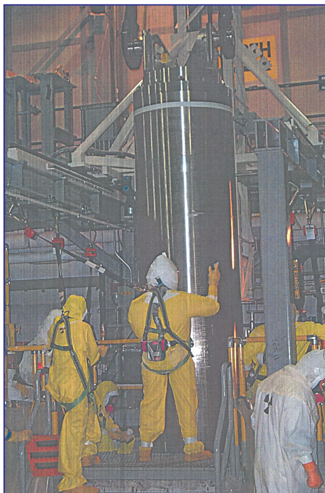
Hanford Site: Spent nuclear fuel project workers moving a Multi-Canister Overpack (MCO) of irradiated fuel From the K-West Basin. The purpose of this project was to move irradiated fuel out of undesirable wet storage near the Columbia River to safe, dry, interim storage in central Hanford. Fuel removal from the K-Basins was completed in FY 2004.
