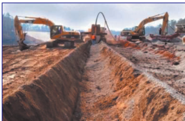
Oak Ridge National Laboratory: Hydrologic isolation activities at the Solid Waste Storage Area 4 (SWSA 4) include employing a state-of-the-art trenching technology that ensures that the project meets the regulatory requirements for reducing groundwater infiltration into the waste burial grounds. Using a one-of-a-kind single-pass trencher, workers are able to install 2,450 feet of continuous pipe and drainage stone at one time. This saves time and has the added safety benefit of eliminating any open trenches. Using laser leveling technology, the trencher automatically adjusts its position to install the 8-inch drainage pipe at the precise depth and slope to divert groundwater around the waste burial ground.
