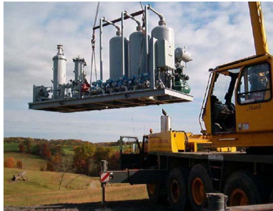
Engelhard's nitrogen removal unit is 8 by 25 feet, with vessels, vacuum pump, instrument air system, valves, and instrumentation. The skid, about 25,000 pounds, is shipped on a double-drop truck and installed by crane.
