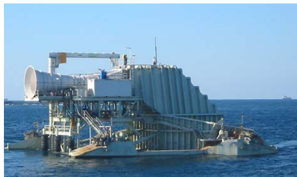
Terminator (Energetech Oscillating Water Column)
