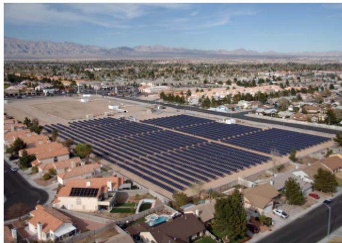
PowerTracker Ground System at the Ronzone Reservoir
