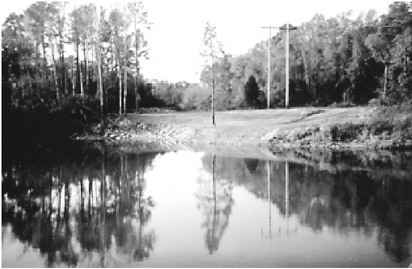
After removal of the Quaker Neck Dam on the Neuse River near Goldsboro, NC.
