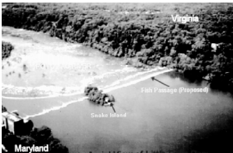
Little Falls Dam on the Potomac River.
