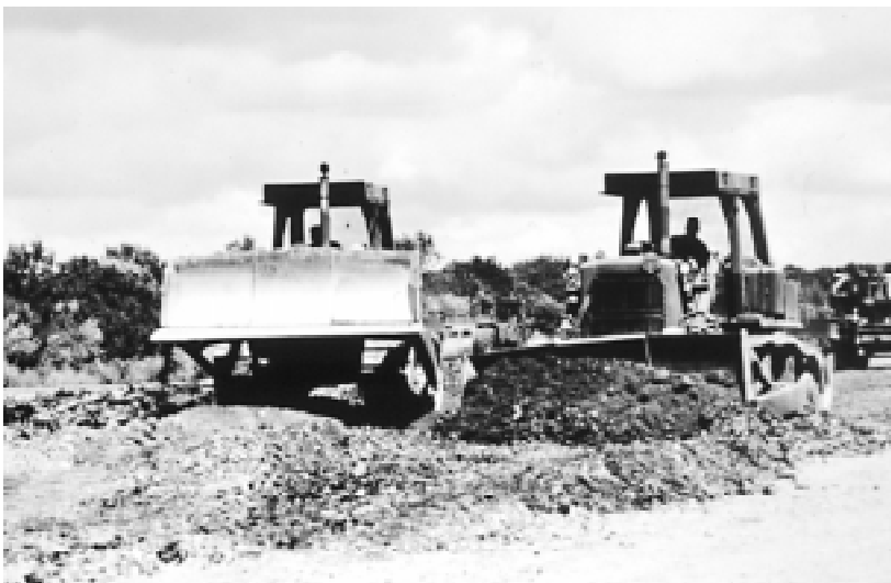
Excavation of asphalt runways by the 368th Construction Battalion, US Army Reserve Unit at the Ninigret Wildlife Refuge, RI.
