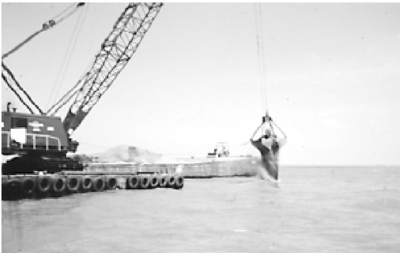
Creation of reefs for oyster spat settlement using fly ash pellets, Galveston Bay, TX.
