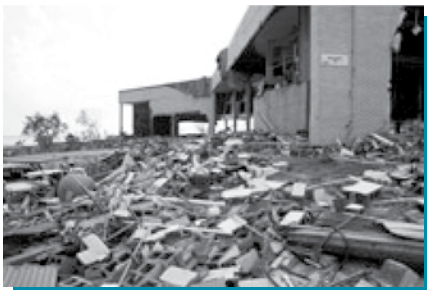
The J.L. Scott Marine Education Center and Aquarium post Hurricane Katrina.
