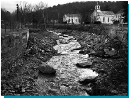
Yokum Brook after the Ballou Dam was removed to restore fish passage.
