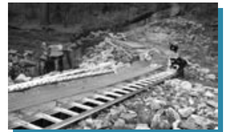
Branford Supply Dam
