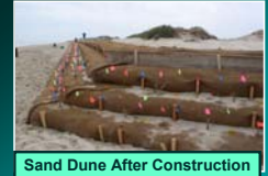
Sand Dune After Construction
