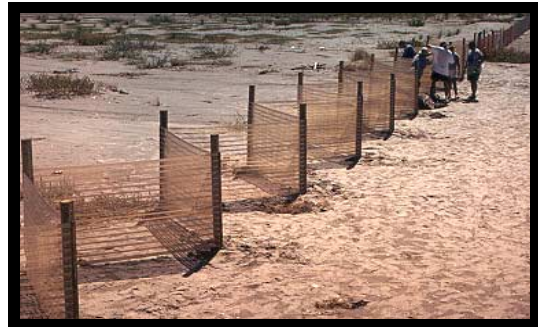
Newly Constructed Sand Fence
