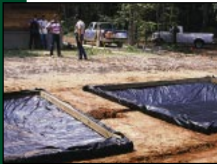
Construction of the ETPMC's wetlands included two lined cells.
