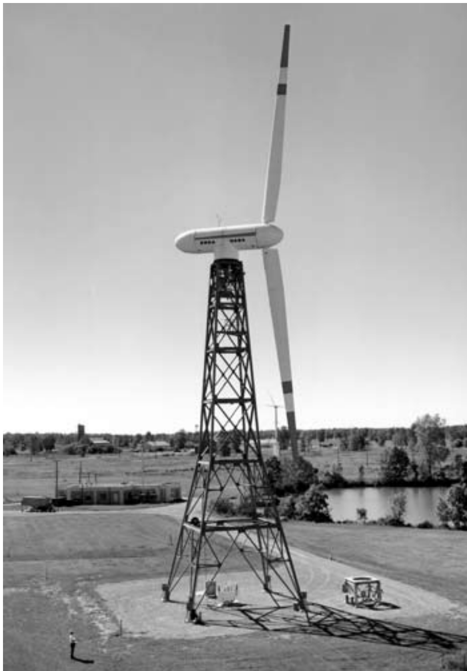
NASA and the Energy Research Development Administration installed this large 100-kilowatt wind turbine for alternative energy research at Plum Brook (28 September 1976). (NASA C-1976-3906)
