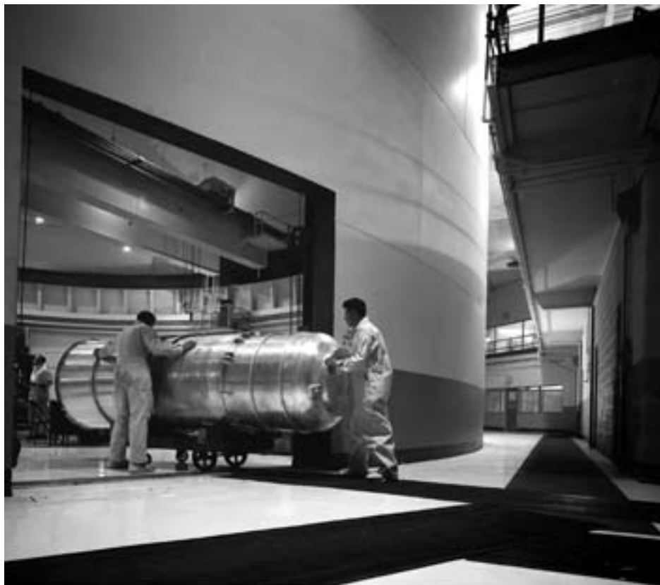
Technicians move a large “thimble” containing experiments for irradiation into the containment vessel. (NASA C-1961-55811)
