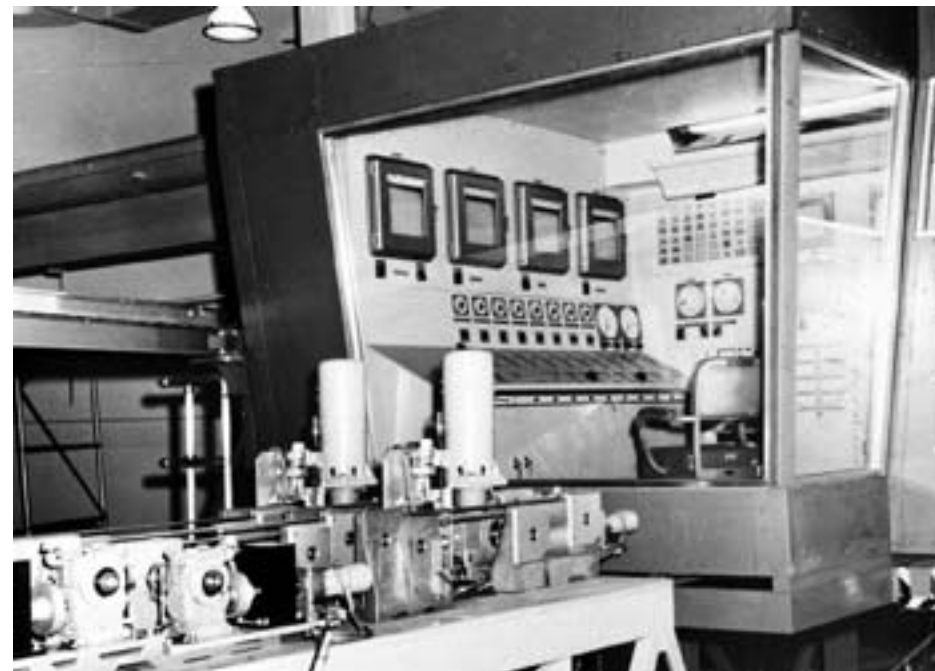
The control room for the Mock-Up Reactor. (NASA PS63-0008)
