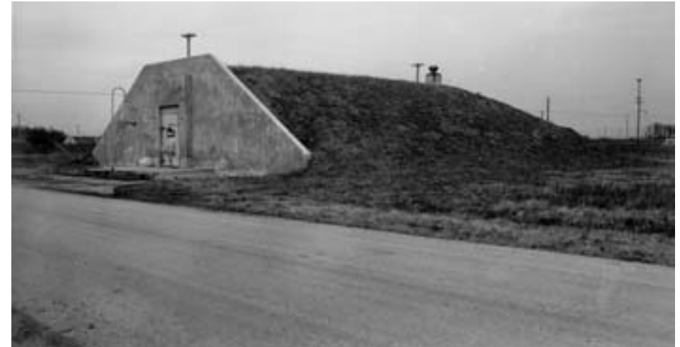
One of 99 bunkers or “igloos” used to store power in Plum Brook’s southwest corner. Courtesy U.S. Army Corps of Engineers, U.S. Army. (No. 21762, 1944)
