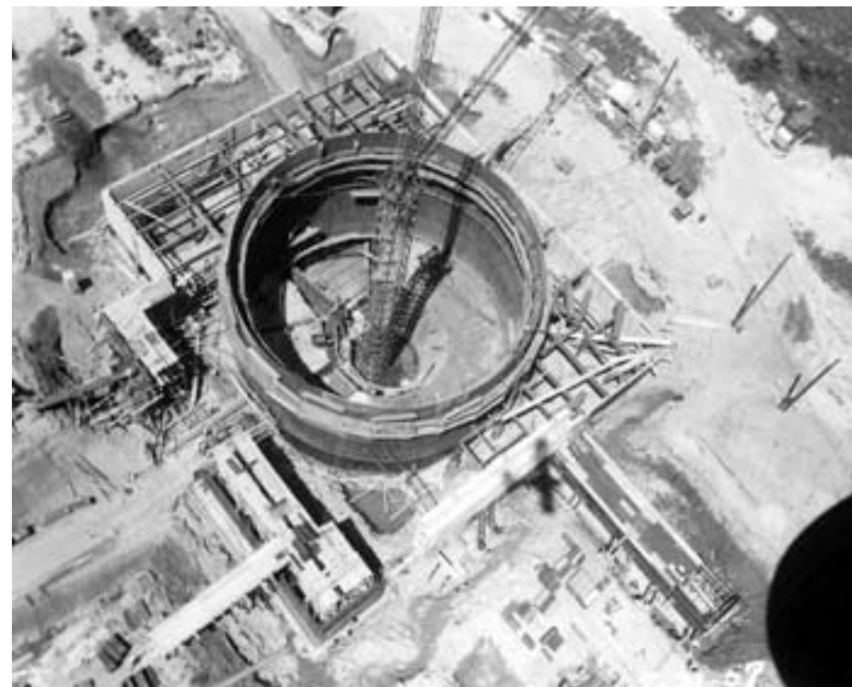
Aerial view of the construction of the containment vessel dome. (NASA 2005-1198)
