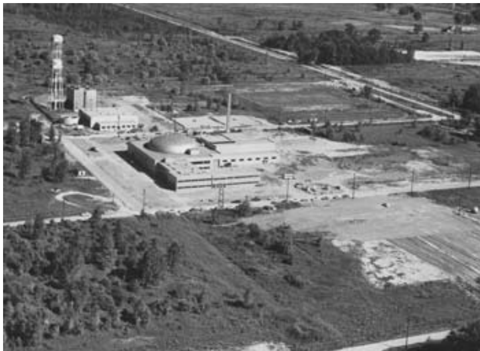
The Plum Brook reactor nearing completion. (NASA 2005-1201)
