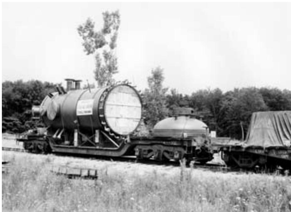
The reactor pressure tank being delivered to Plum Brook by railroad. (NASA C-2003-833)
