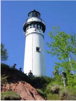
Outer Island Lighthouse
