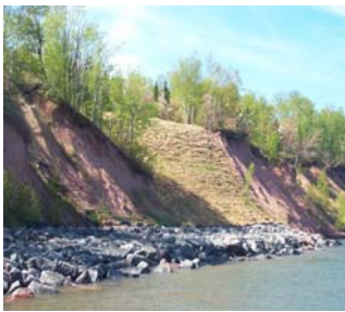
Newly seeded and mulched slope
