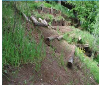
Establishing slope grid and vegetative cribwalls
