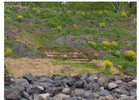
Crib wall on Raspberry Island starting to grow and establish
