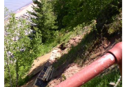
Established crib wall on Outer Island
