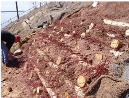
Newly constructed crib wall on Raspberry Island
