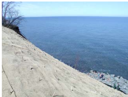
Live stakes on newly graded, netted, steep slope on Outer Island
