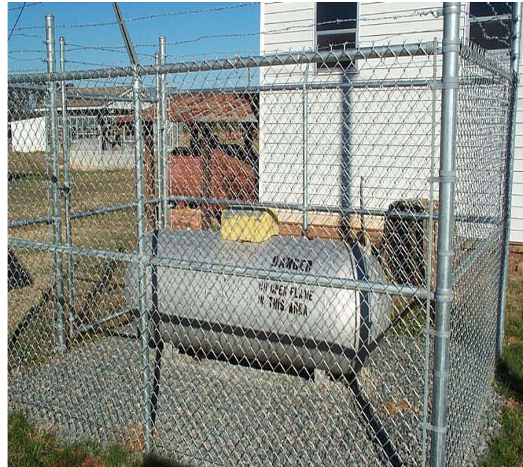
New Propane Tank Fences
