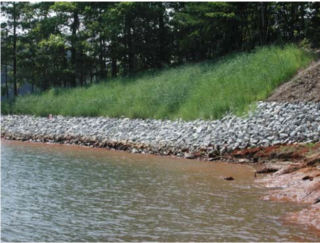
Streambank Stabilization (Alamo switchgrass)
