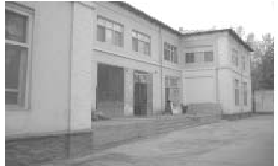
The "Yellow House" construction renovation project where OIG found a $57,605 double-billing, plus indirect costs. The building was never used by the contractor and was turned over to the Afghan government.
