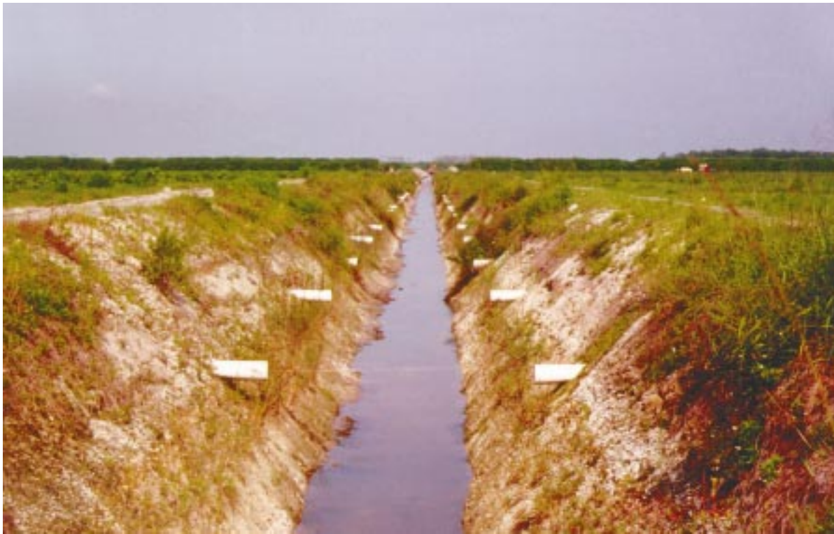
Figure 4. Drainage canal with furrow drain pipes extending out of the wall of the canal, St. Lucie County, Fla.
