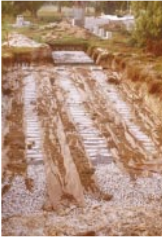
Installation of septic tank and drain field in southern Florida.
