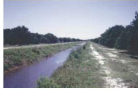
Drainage canal in St. Lucie County.
