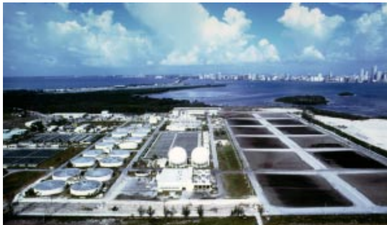
Domestic wastewater facility, Dade County. (Photo courtesy of the Florida Department of Environmental Protection.)
