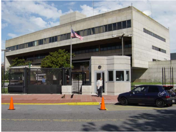
Exterior of Embassy Buenos Aires
