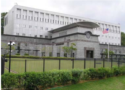
Exterior photograph of Embassy Singapore
