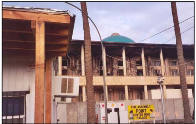
Partially destroyed Embassy Baghdad communications center
