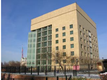
Exterior of Embassy Moscow
